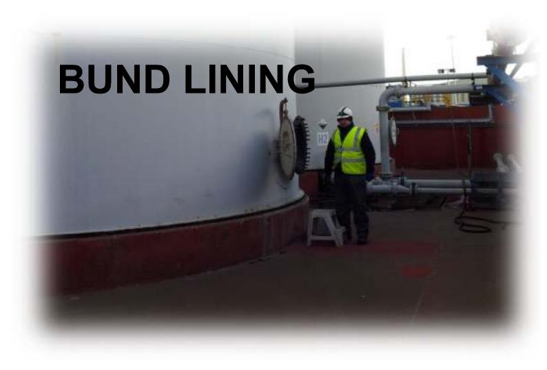
Effective bunds should be in good repair, of adequate size and completely watertight.
